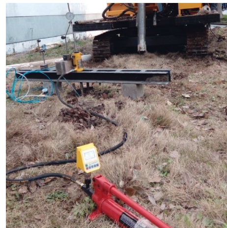
FIGURE 10: Field test set-up.
